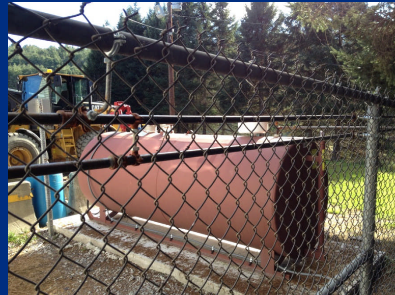
New above-ground tank
