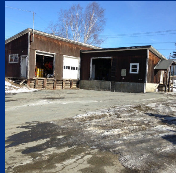
Store keepers office and cold storage (existing)
