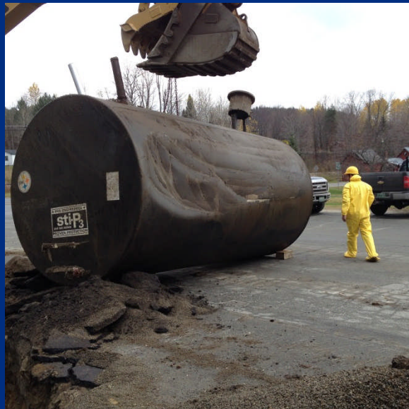
Removal of old tank
