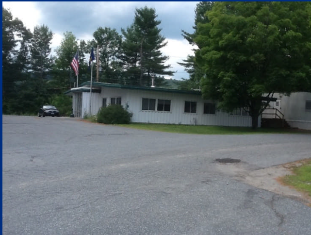
Office Building (existing)
